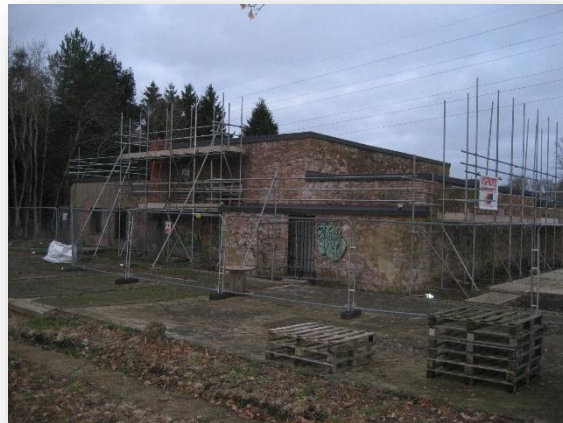
Figure 10: Building at Former Grafton Underwood Air Base
