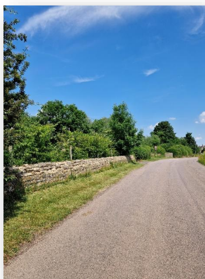
Figure 8: A local boundary wall
