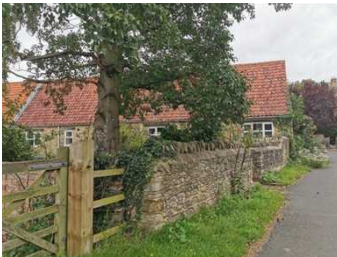
Figure 29: Low limestone rubble wall
