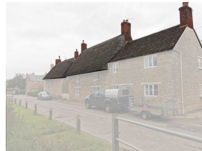
Figure 28: Open gable roof
