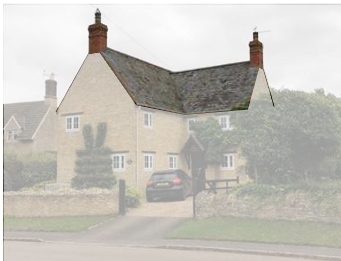
Figure 27: Cross gabled roof
