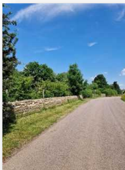
Figure 8: A local boundary wall
