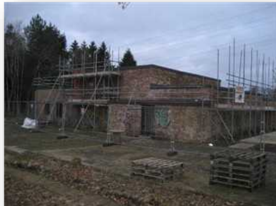
Figure 10: Building at Former Grafton Underwood Air Base
