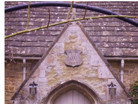
Former School: roof details
