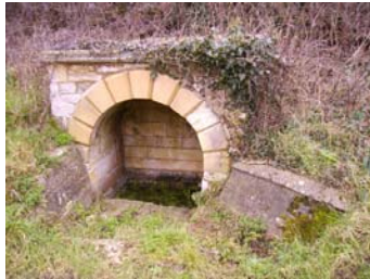
Well Head, Geddington Road
