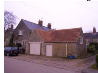
No. 26 Former Workshop
